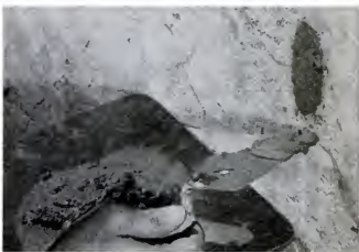
Fill holes solidly with a 1-to-2 mortar mix.
